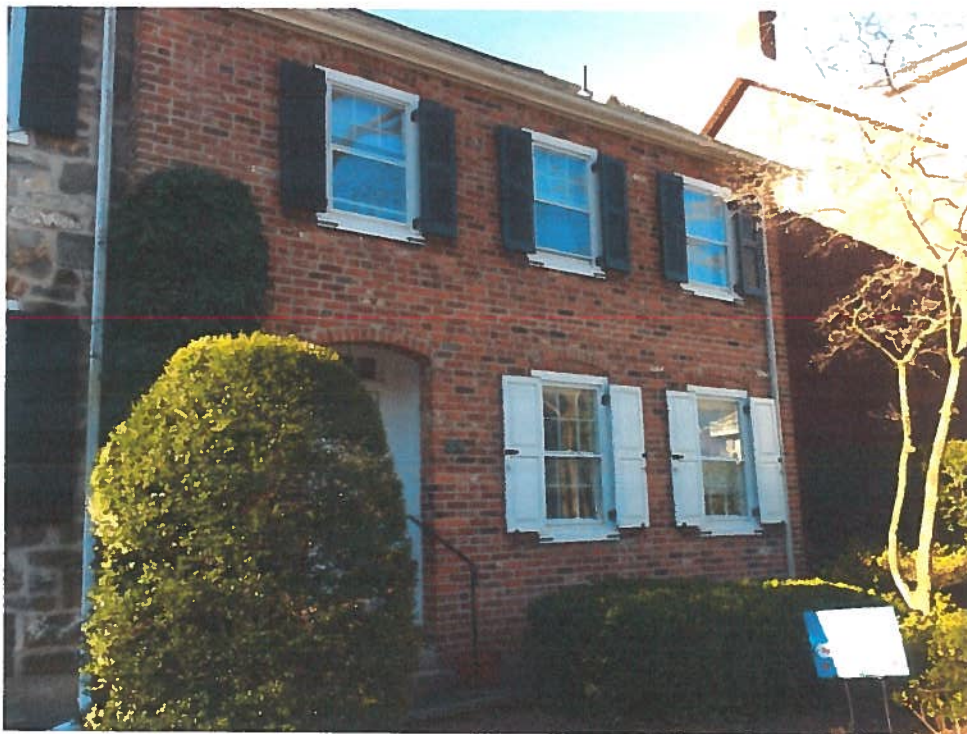
Figure 3. 52 E Wall St – recently installed Western Red Cedar Shutters. The “top black” / “bottom white” shutter motif only occurs on the two brick end-unit townhouses.
