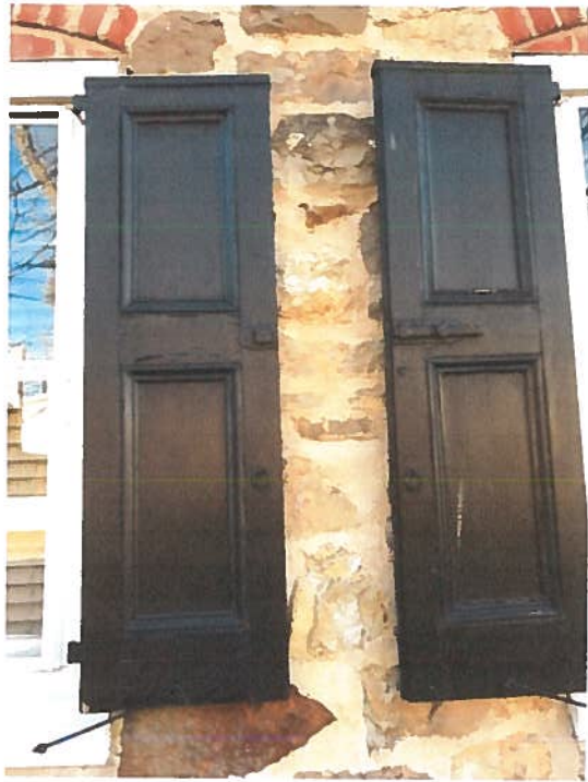
Figure 6. Existing Ground Floor Shutters at 54 E Wall St. – Flat Panel Shutters
